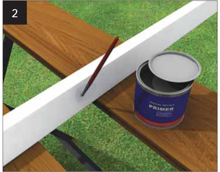
2 Ensure the surface is dry – apply a thin primer coat using a fine brush.
