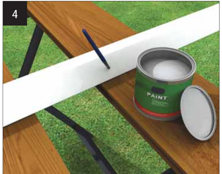
4 Finally, apply an air drying top coat with a fine brush.
