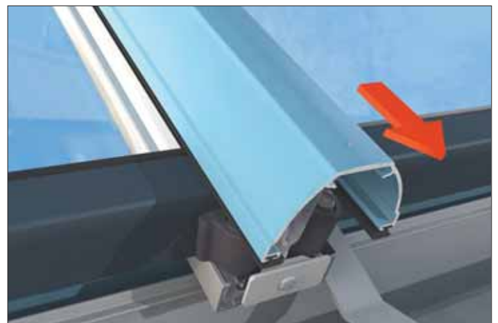
Slide the end cap up and off the fixing block and unscrew the fixing at the end of the glazing bar (reverse steps 05 and 06). Slide the glazing bar top cap down to release it from the spring loaded clip. To re-install repeat steps 1-6.
