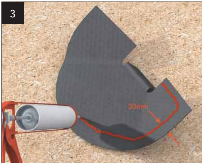
Apply Gutterbond supplied to underside of flashing.
